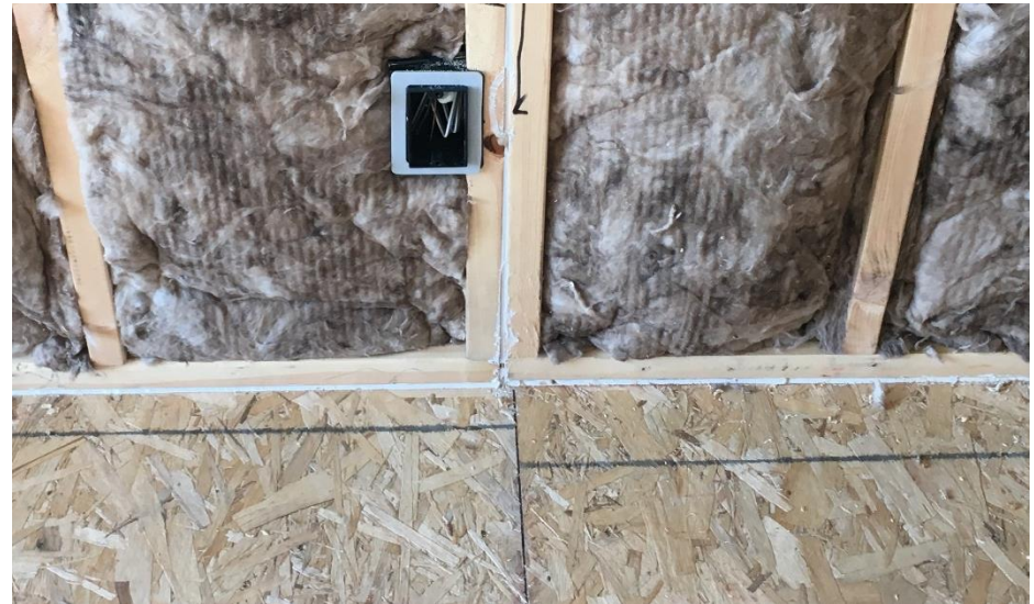
Caulk at sill plate
