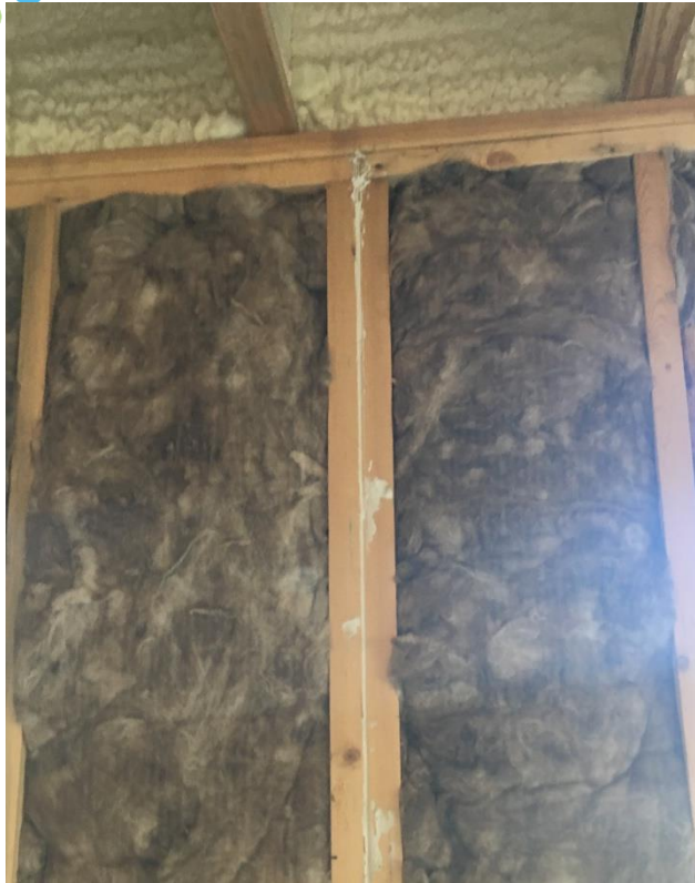
Caulk at seams where wood is joined
