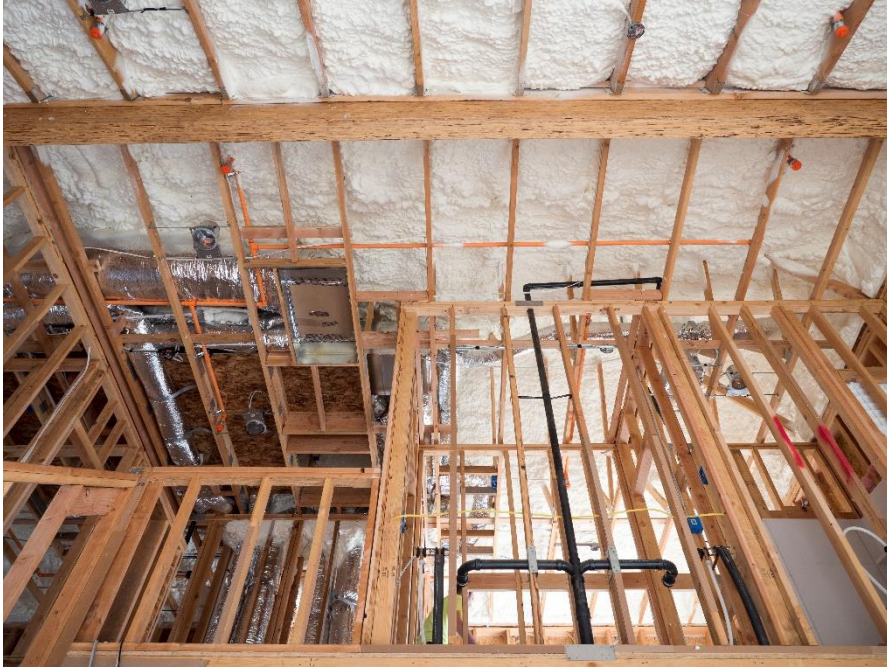
Foam at roof deck
