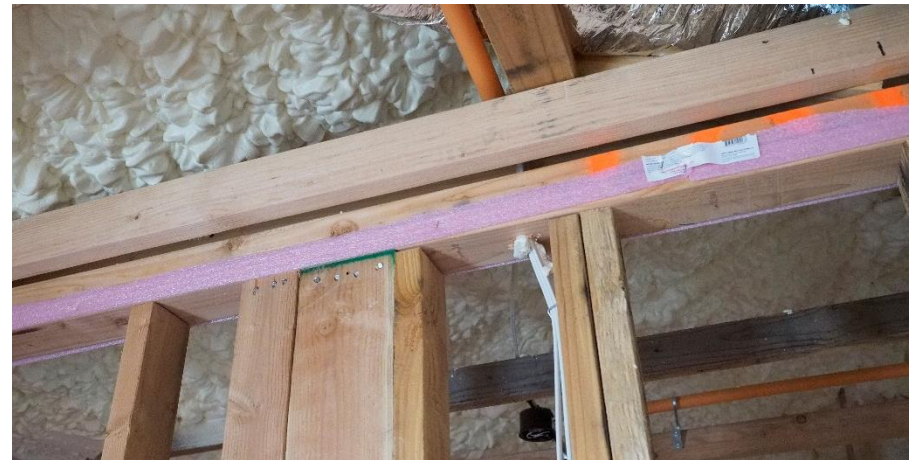
Foam gasket to seal drywall to top plate
