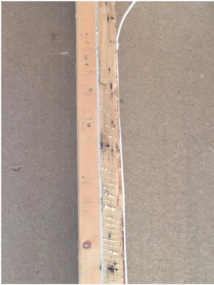
Seal formed between studs
