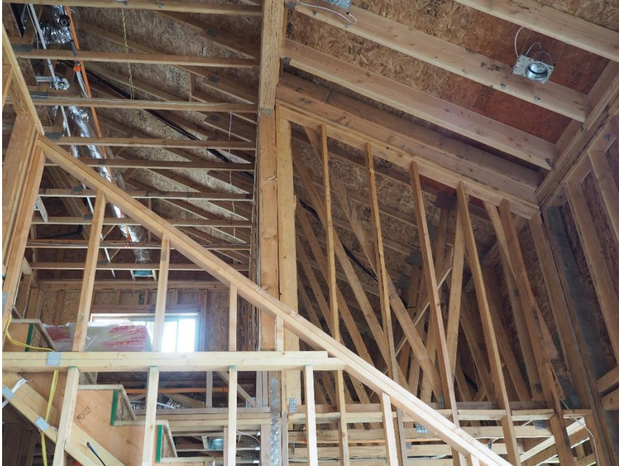
Exposed roof deck
