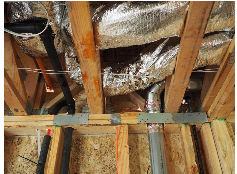
Rim joist penetrations
