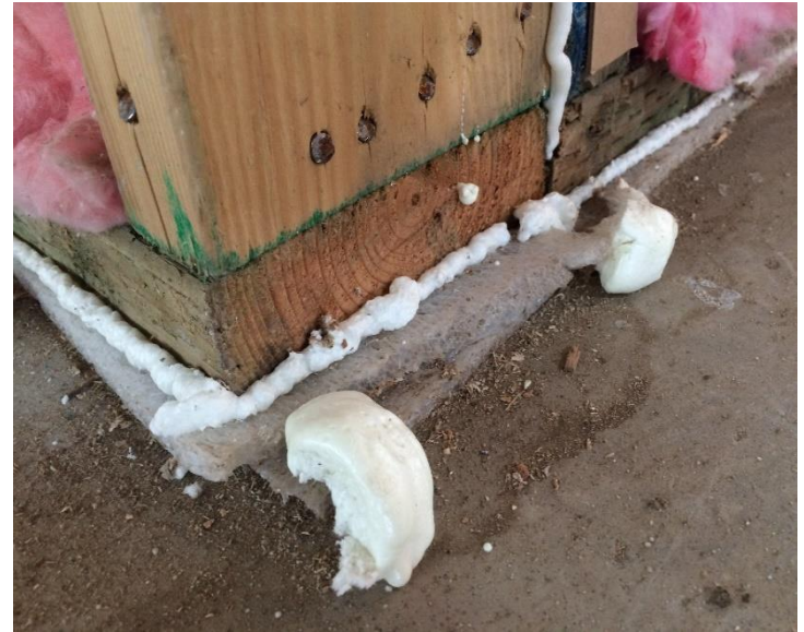
Can foam and gasket at sill plate
