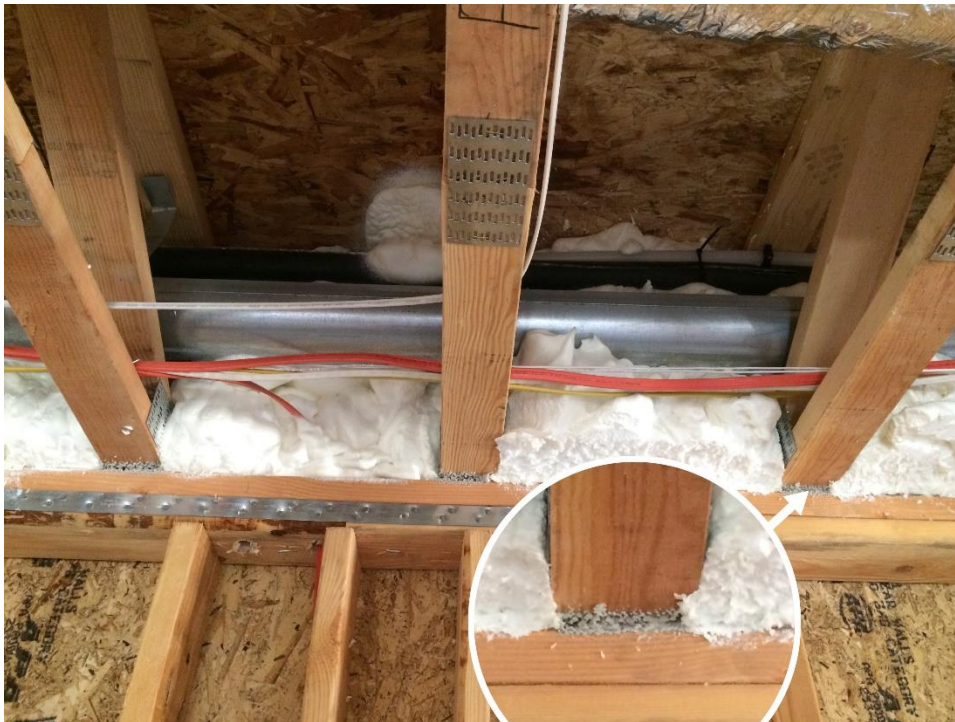
Seals formed under trusses
