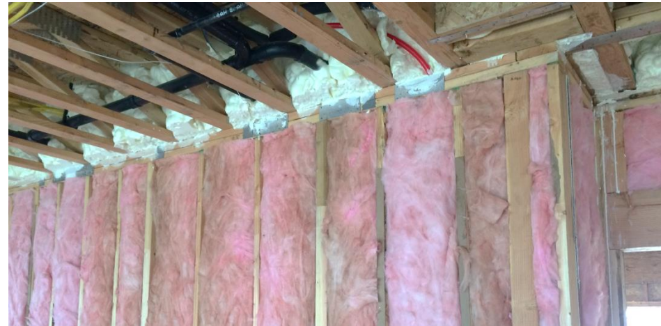
Foam at rim joist
