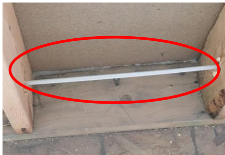
Bottom plate/sheathing gap
