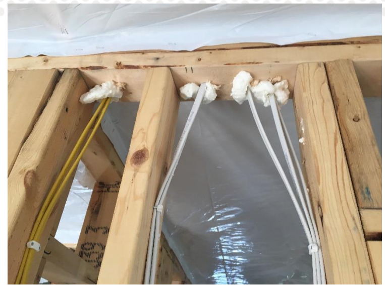
Can foam at wire penetrations
